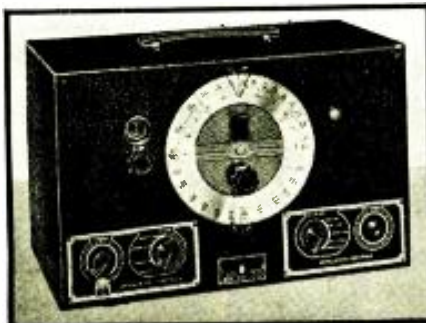
Fig. B. This signal generator has 0.5% accuracy.
